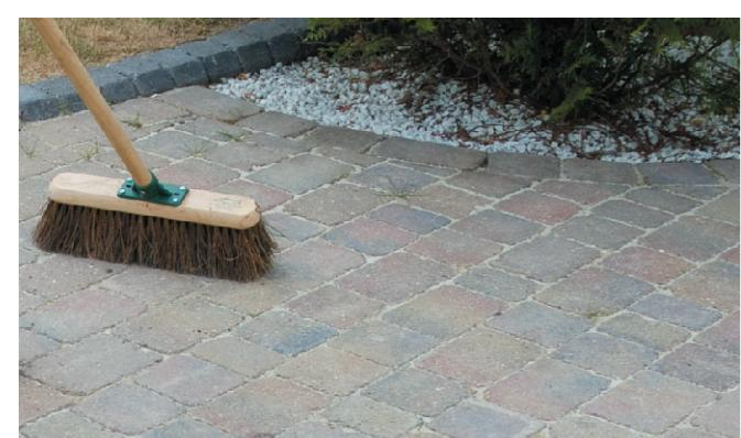
Use of equipment that vacuums or water blasts the paving may remove large amounts of Jointing Sand, reducing the structural integrity of the installation.
