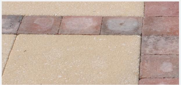
Efflorescence is an unpredictable, but temporary, process. Once all the salt from the paving has risen to the surface it is commonly worn away through use or by weathering. This process seldom takes more than 12 months.
