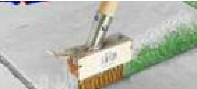
Remove moss, grass and other debris or vegetation from the joints using a proprietary wire brush.
