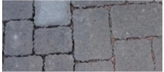
The joints on the right are full, whereas the joints on the left require topping up with new joint aggregate.
