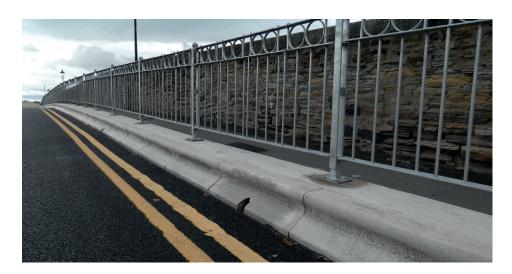
This design feature would prevent the guard rail being used as a lever to pop the kerbs out of position if hit by large vehicles.
