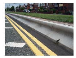
on the lower carriageway and Trief Cadet GST1A on the upper to level the central verge. Access points were built in so that the lanes could remain live and access was designed at each end of the verge runs to enable the mowers to move from one part of the verge to the next.
