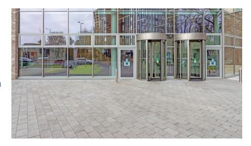
Our AggTech process uses unique natural aggregates on the surface of each paving block to create a stunning durable finish perfectly replicating natural stone. The paving was delivered in four complementary colours - Pearl, Moonstone, Onyx, and Citrine - in a 300x200 paving layout design plan.
