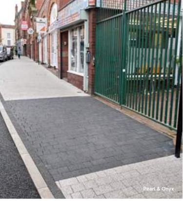
This required bedding in mortar to take up the differences in the depth of the blocks.
