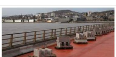
figure was 1.795 kN per metre of kerb therefore Brett Landscaping provided bespoke kerbs which were a maximum width of 336mm to enable the units to be below the required mass. This solution prevented the need to narrow lanes, thereby maintaining optimal traffic flow and safety on this heavily trafficked route in and out of Dundee.
