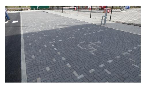
the landside logistic developments of the port which would withstand the damaging effects placed on the pavements with the constant trafficking of heavy goods vehicles. Rectangular block paving also provides a surface which has a lower whole life cost than using other surfacing materials due to the ease of reinstatement and maintenance throughout the pavement's lifetime.
