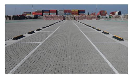
greater rigidity of the pavement surface compared to standard rectangular block paving.
